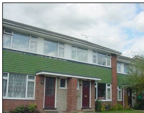
1960s/1970s cross wall construction
