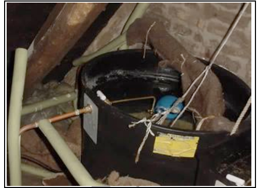
Un-insulated water tank
