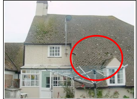
Rear cap slide roof
