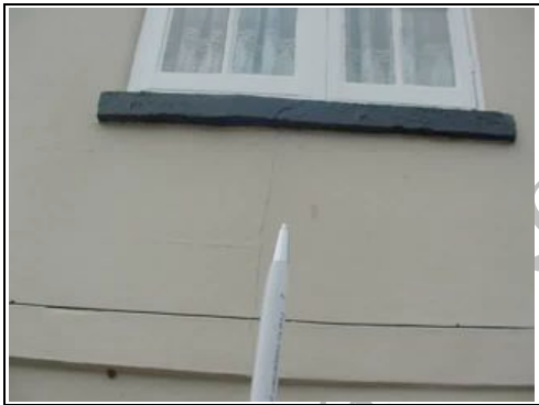
Cracks in render
