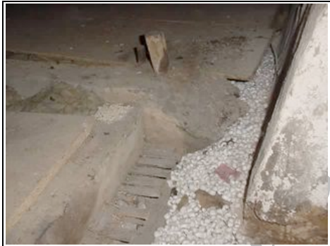
Spine beam that does not tie in
