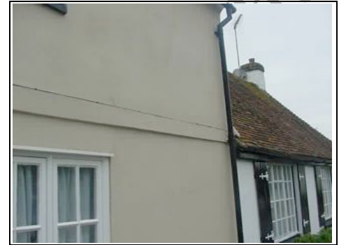
Painted cement rendered walls covering timber frame
