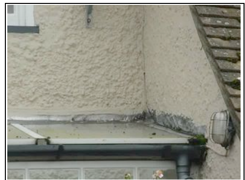
Poor detailing to rear low level roof
