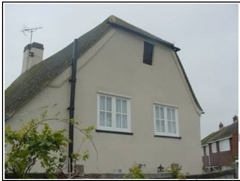
Thickening of the render at high level
