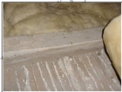
Lath and plaster ceiling
