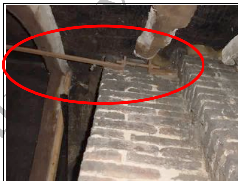
Bracing running from front to rear
