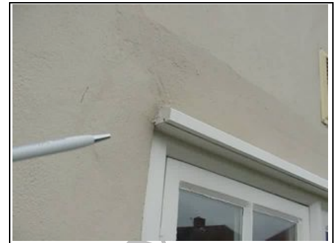
Drip detail to window
