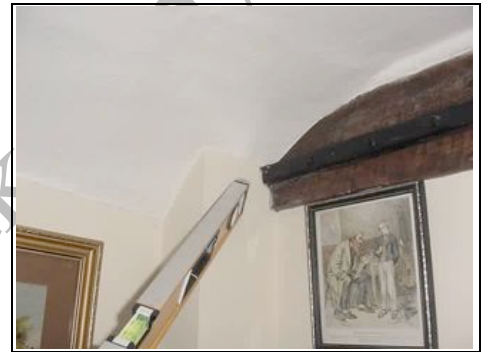
Bracing straps
