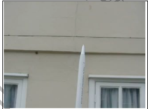
Cracking to render
