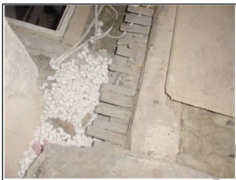
Lath in ceiling overclad
