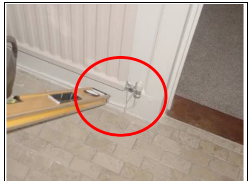
Micro-bore pipes
