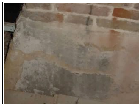
Dampness to chimney breast in roof
