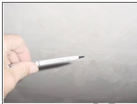
Hairline cracking
