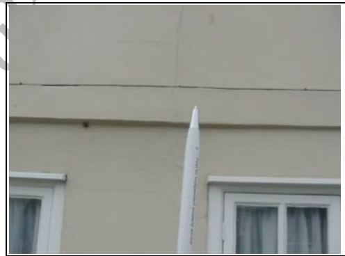
Cracking to render
