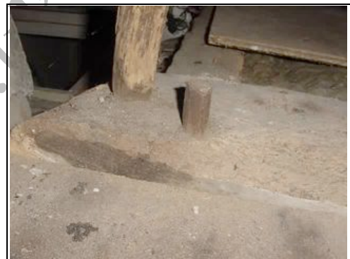
Peg fixing spine beam not tied in
