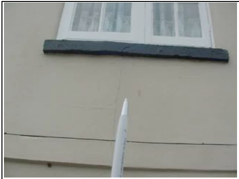
Cracks in render
