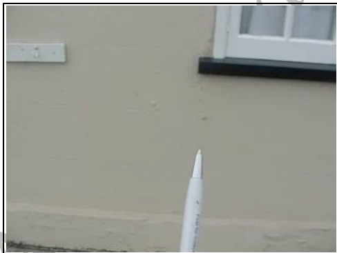
Cracking occurring to render
