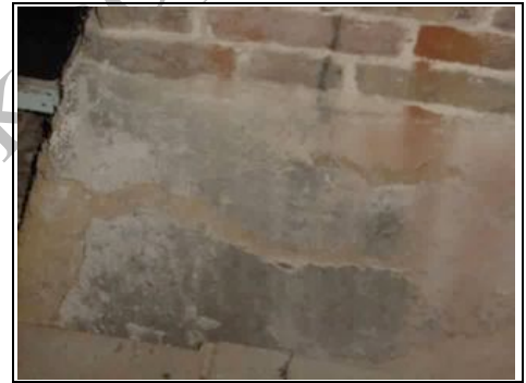
Damp plaster to chimney breast
