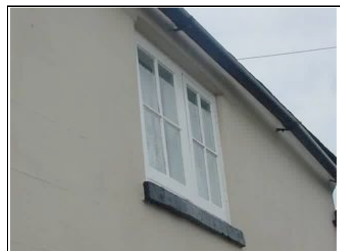
Render has cracking
