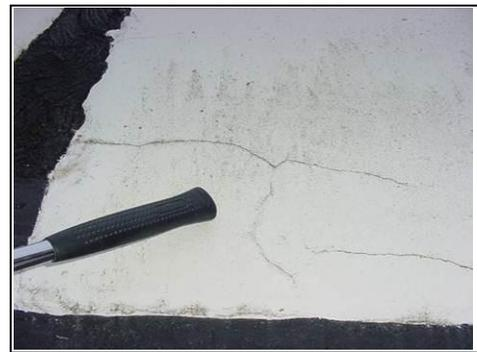
Loose render around the cracking
