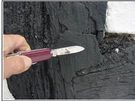
Plastic wood repairs to the timber structure
