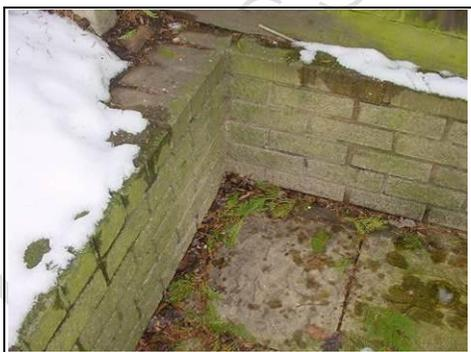
Small retaining walls need weep holes
