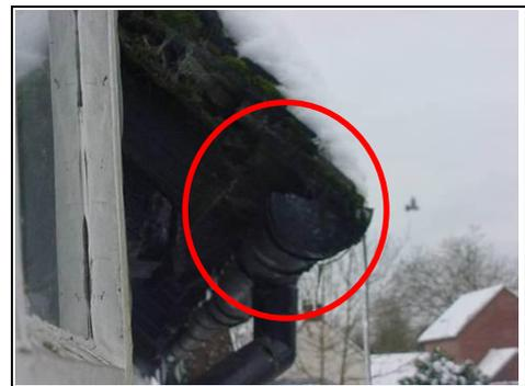
Guttering out of alignment
