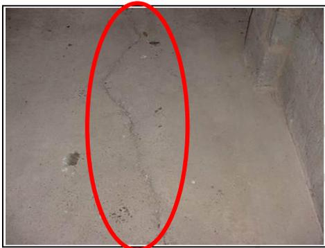
Crack in the floor follows the line of the building
