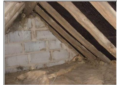
Blockwork visible in the roof space right hand side.
