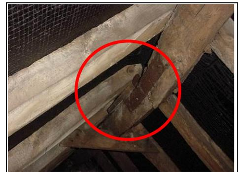
Metal bracket added to broken ridge timber
