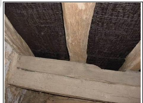
This photo shows the common rafters in the left hand side (the ones that form the pitch of the roof) and the dark area between is the underlayer
