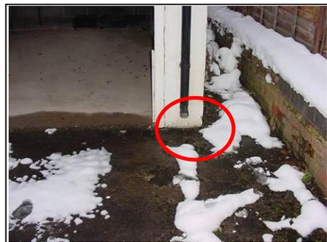
Gutters discharging onto the ground
