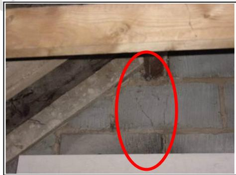
Crack can be seen in the block work
