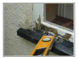
Rotting window due to there being no drip detail above and the quality of timber is not that good
