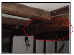
Spine beam has been cut away to increase head room on the old staircase
