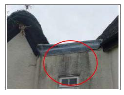
Pattern staining to the rear of the property due to the lack of detail
