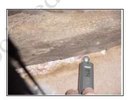
High reading of 74 to the stone/tile below the sole plate explains the rot
