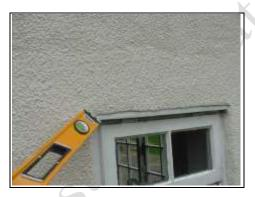
The original drip in the wood has been lost due to the render
