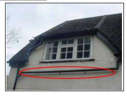
Eyebrow roofs make it awkward to run the guttering Very horizontal downpipe (red)
