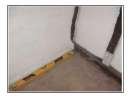
Sole plate not visible to left hand side -level indicates where it should be
