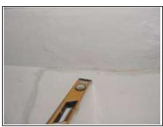
Cracking to small bedroom in older building travels between the wall and the ceiling
