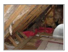
Cut timber roof with props added, often after roof spread
