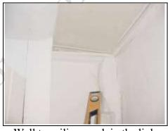
Wall to ceiling crack in the link corridor, first floor
