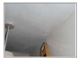
Cracking where the old building meets the new
