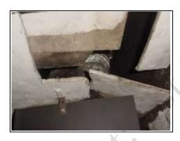
Possible asbestos in the chimney
