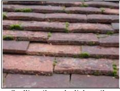
Spalling tiles – the lighter tiles
