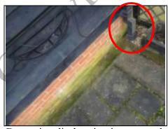
Downpipe discharging into ground, we would expect it to discharge into a soak-away
