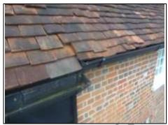
Bolts projecting on the gutters which makes the gutters block up, need to be made flush
