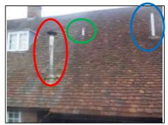
Metal flue (red oval), small flue to middle is from an extract fan (green oval) and soil and vent pipe (blue oval)
