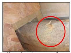
Signs of woodworm to purlin on right side of roof
