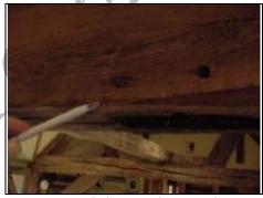
Two peg joints on beam where brace is missing
