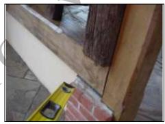
Honest repair in original timbers which stand out and what looks to be newer brickwork
