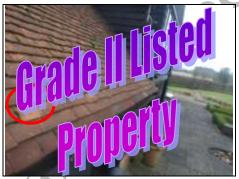
Close up of spalling tiles and moss on roof Aerial view – 360 photo
