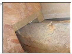
Woodworm and softness in rear right purlin in right roof void
