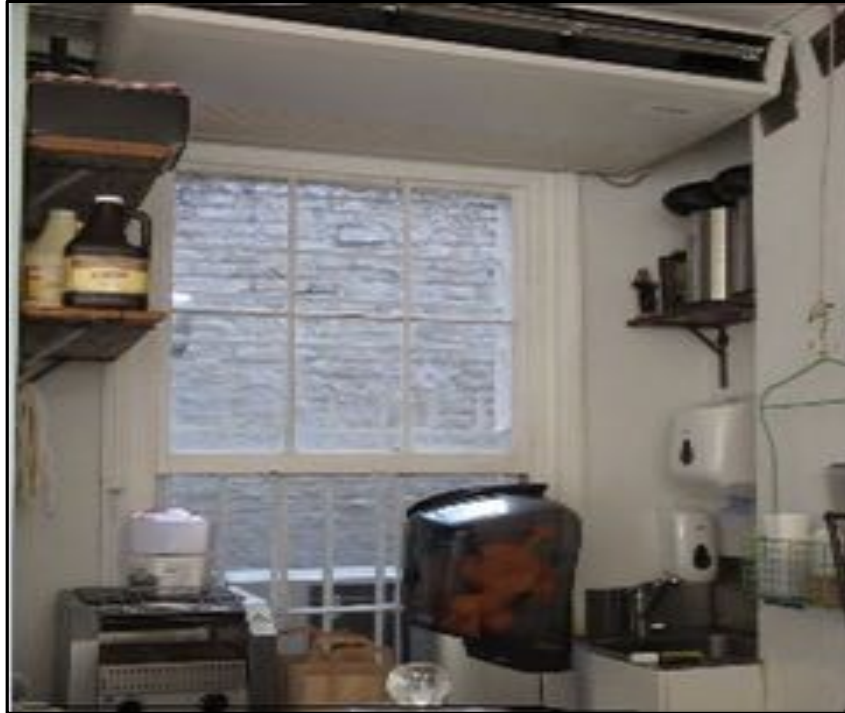
Original Vertical Sliding Sash Window at rear of premises (XXXX Author)
