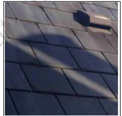
Vent on main/loft conversion roof
