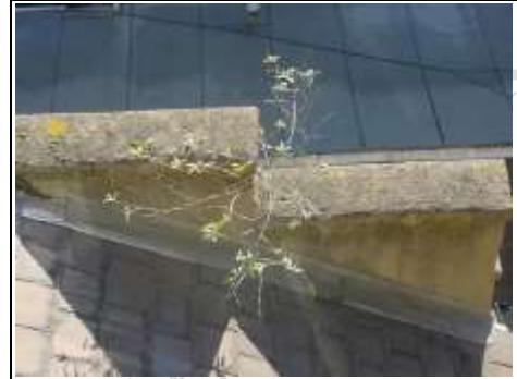
Rear parapet wall/balustrade without box gutter detail. Plants growing from it indicate that dampness is getting in to it
