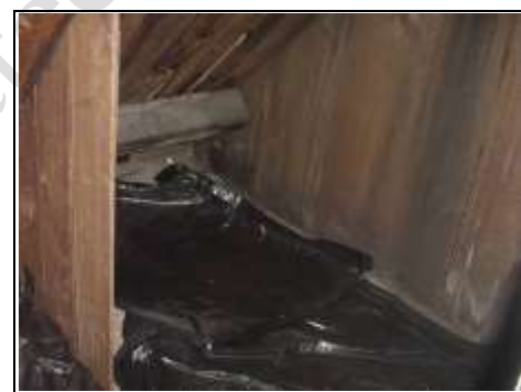
Dampness getting into roof on fifth floor
