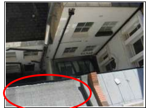
Your patched mineral felt roof to left hand side is in poor condition compared with next door's lead finished roof to the right
