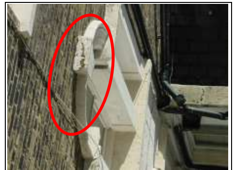
Dampness to the mouldings around the window and the keystone where there is a ledge
