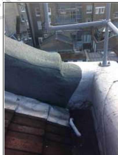
Mineral felt to rear parapet wall
