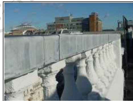
Lead capping to front balustrade
