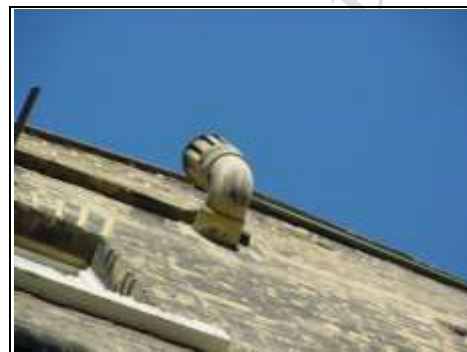
Asbestos flue to rear
