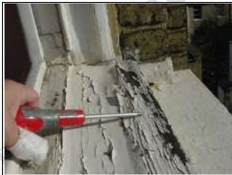
Timbers deteriorating
