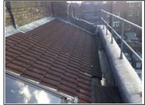
Single pitched concrete tiled roof
