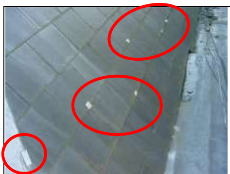
The light coloured clips are the lead tingles to loft conversion roof on the right hand side
