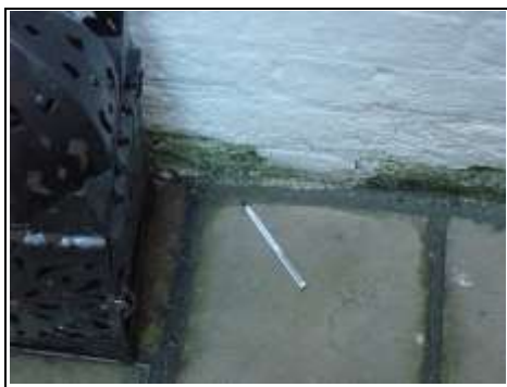
Tiled floor with areas of mould
