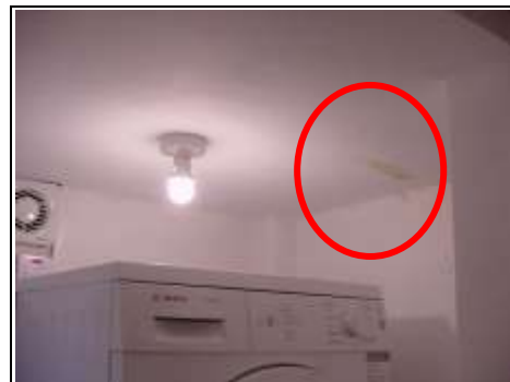
Staining on ceiling in utilities room on lower ground floor
