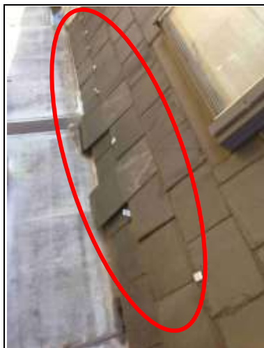
Left hand view of roof; far too many lead tingles and slates completely slipped
