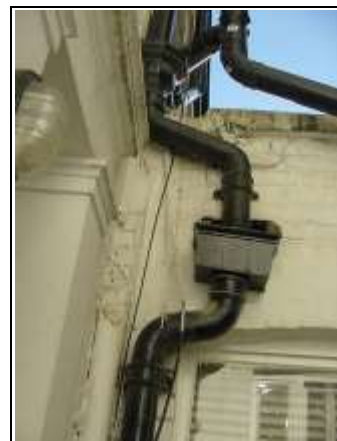
Cast iron hopper head
