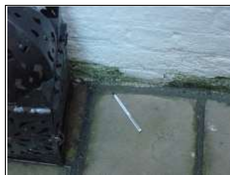
Painted brickwork to rear with areas of mould to the base
