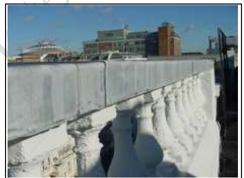
Balustrade/parapet to front with its own capping
