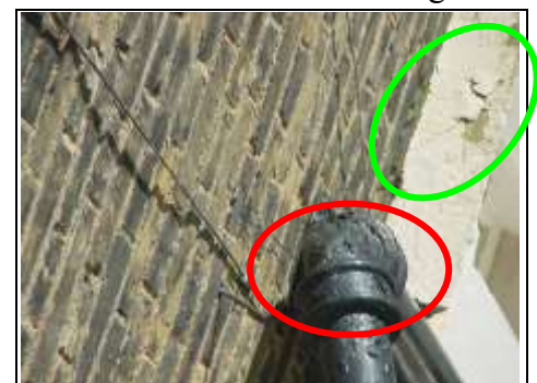
Cast iron pipe (red circle) and moulding (green circle) in need of redecoration
