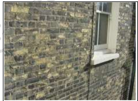
Flemish Bond brickwork at high level
