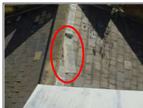
Lead flashing coming away on rear single pitched roof to your side
