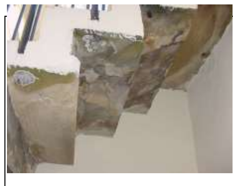
Underside of steps showing water getting through
