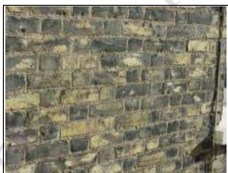
Rear brickwork where ad hoc repointing is needed
