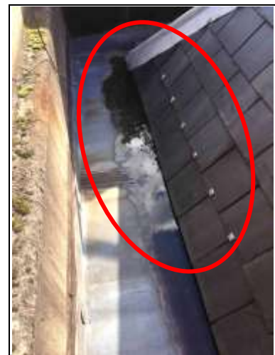
Rear left hand corner – more lead tingles and also ponding within the box gutter
