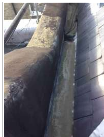
Bitumen covered parapet wall
