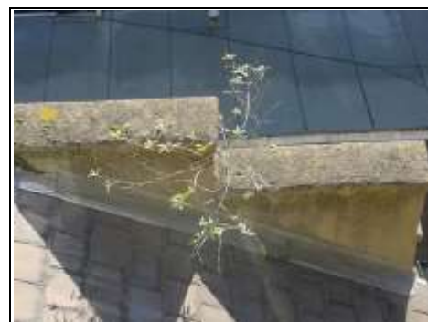
Plant growing out of parapet wall
