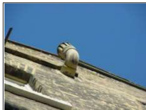
Asbestos flue to rear
