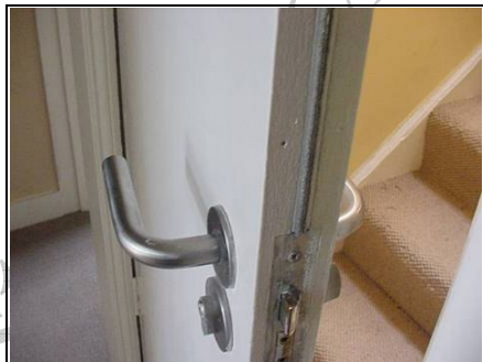
Fire door to entrance to top floor with intumescent strip
