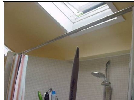
Pen indicates hairline cracks in top floor ceiling, again likely to relate to plasterboard
