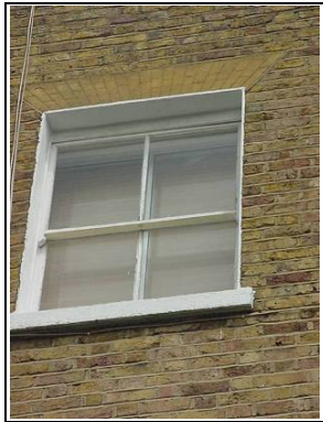
Close up of top floor sliding sash window
