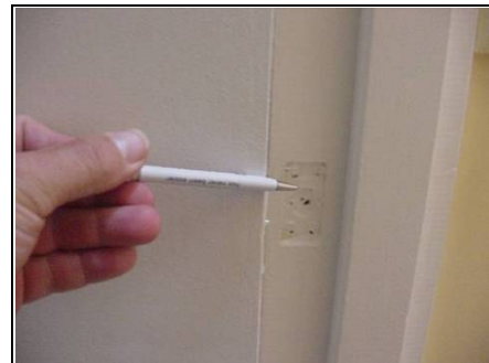
Perco fire door closer removed
