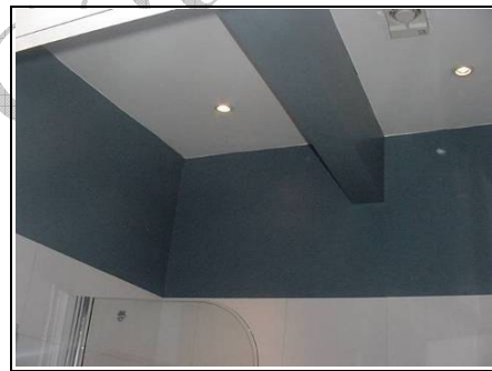
Ceiling in central bathroom on first floor – there are leaks in the ceiling, likely to be modern plasterboard
