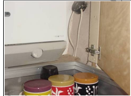
Potterton profile wall mounted boiler
