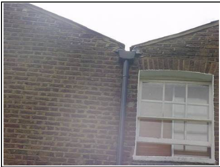
Plastic hopper head and downpipe from the main butterfly roof
