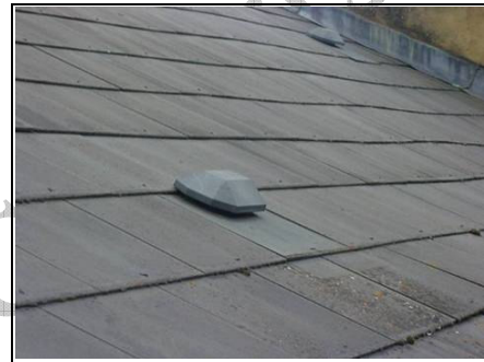
Air vent on roof
