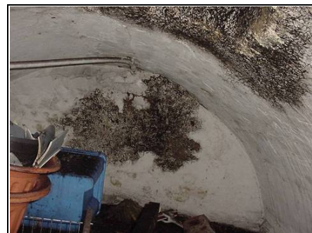
Possible fruiting body of dry rot in lower ground floor
