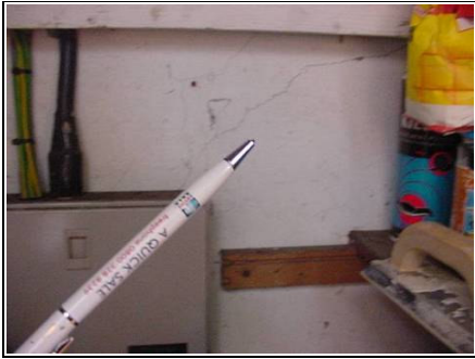
Cracking under stairs
