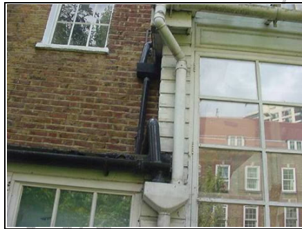
Gutters and downpipes from the conservatory roof
