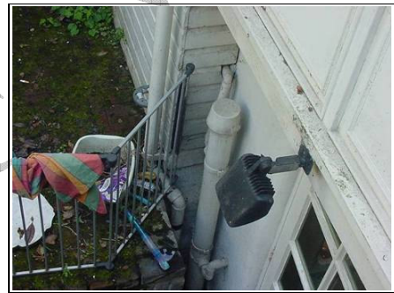
Dergo valve or soil and vent pipe between lower ground and upper ground floors
