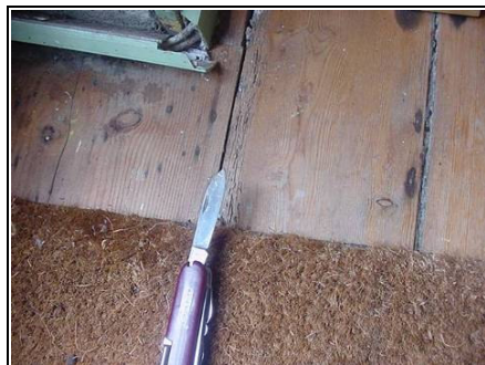
Old woodworm in lower ground floor
