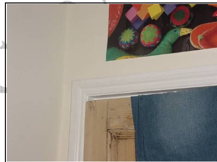
Rear bedroom where movement can be seen in the door frame
