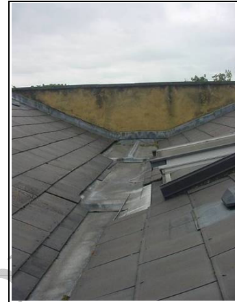
Parapet wall and stepped valley gutter
