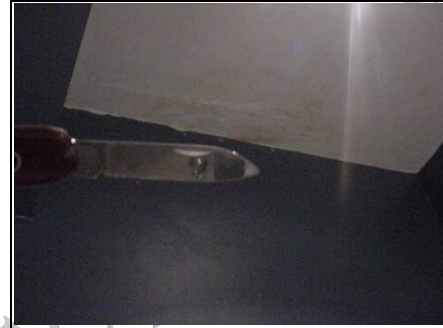
Knife indicates water damage on bathroom ceiling below
