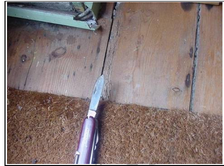
Signs of old woodworm on lower ground floor
