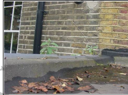
Leaking flat roof
