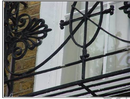
Cast iron in front of window rusting slightly
