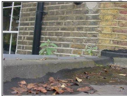
Leaking flat roof covered with moss
