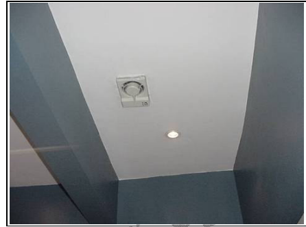
Extract fan first floor bathroom does not work
