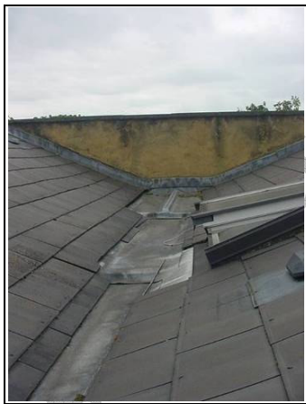
Butterfly roof with stepped valley gutter
