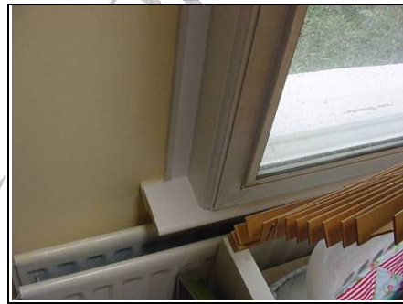
Good quality secondary glazing on the top floor
