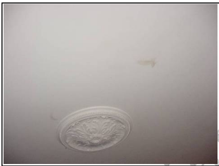
Ceiling rose lower ground floor, possibly original lath and plaster
