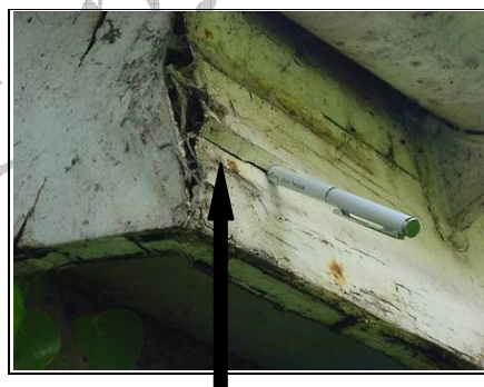
Pen pushing into deteriorating fascias and soffits
