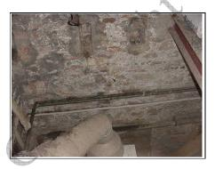
Asbestos going down to boiler in handyman's room and boiler room
