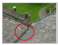
Valley gutter that is becoming blocked next to a lead guttering
