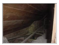
Far left hand side – here you can see a timber decking has been used to support the valley gutter which looks in reasonable condition
